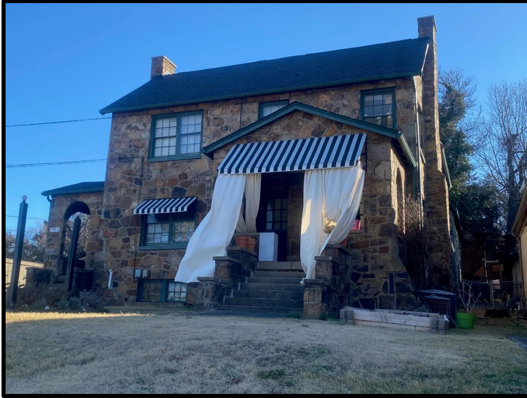
Figure 54. 1160 N College Ave building (facing east)
