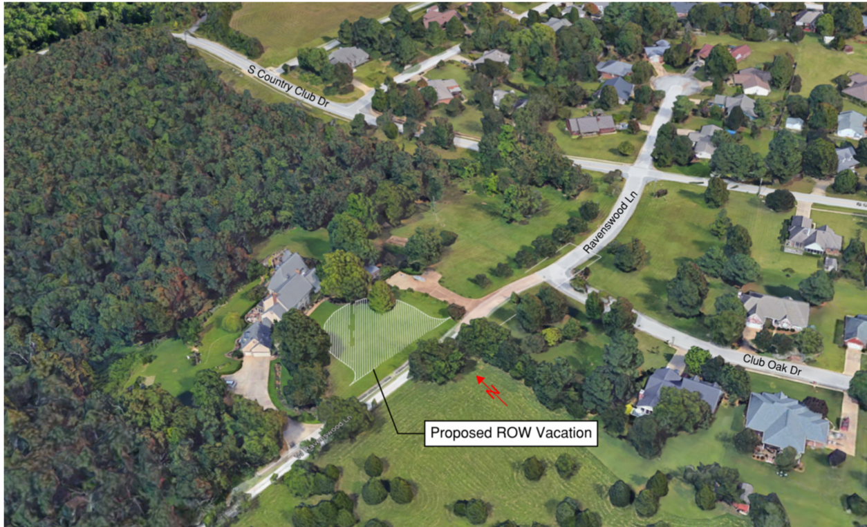
Exhibit 2: Aerial image of proposed right-of-way/front lawn of subject parcel.
