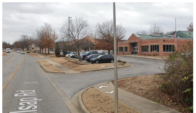
EXISTING SIDEWALK SYSTEM
