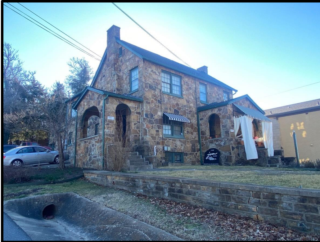
Figure 56. 1160 N College Ave building (facing southeast)
