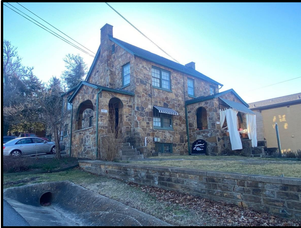
Figure 56. 1160 N College Ave building (facing southeast)
