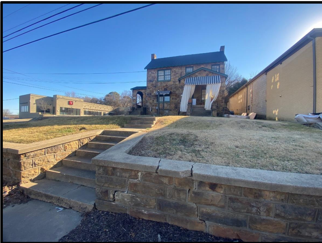
Figure 55. 1160 N College Ave building (facing northeast)
