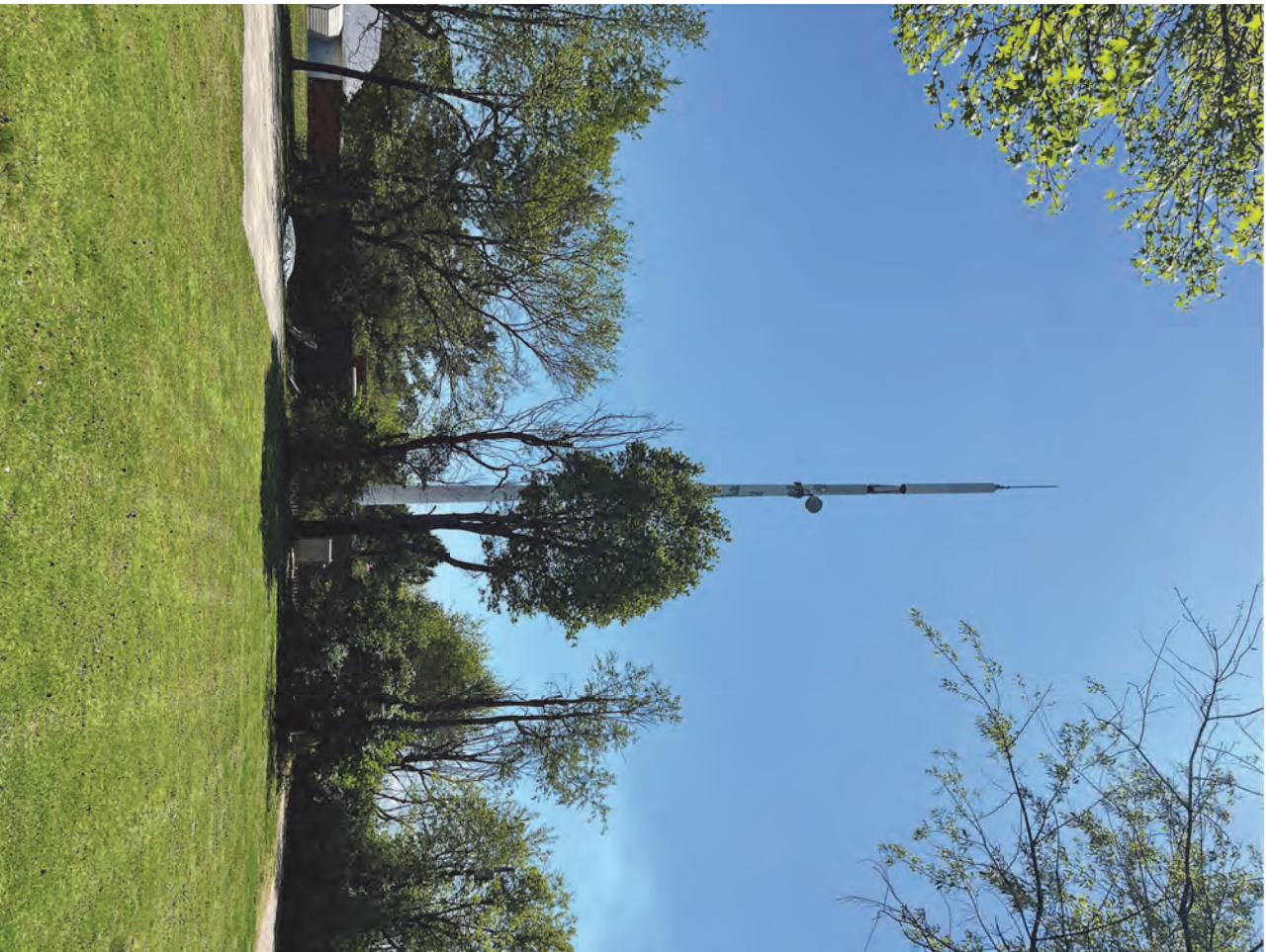
Location G - Existing tower - North @ 150'
