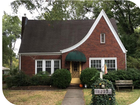
Historic Resources Survey Update of the Hendrix College Addition NRHP District Conway
