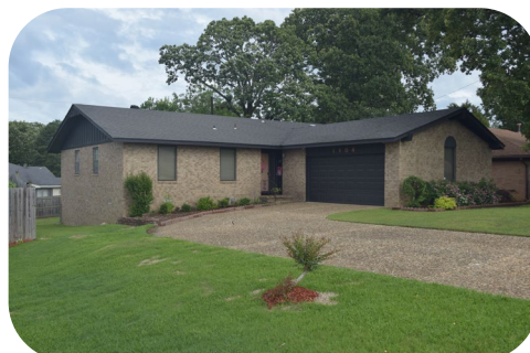
Historic Resources Survey and NRHP Nomination of University Park Little Rock
