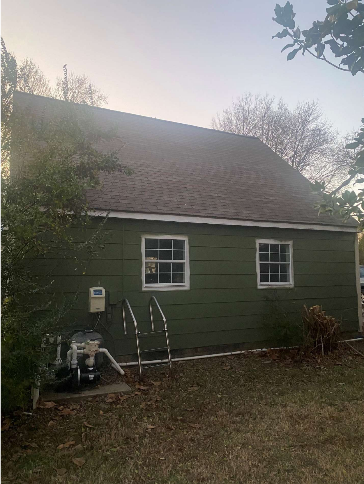
Elevation View of Exterior
