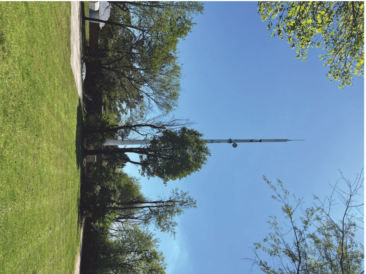
Location G - Existing tower - North @ 150'
