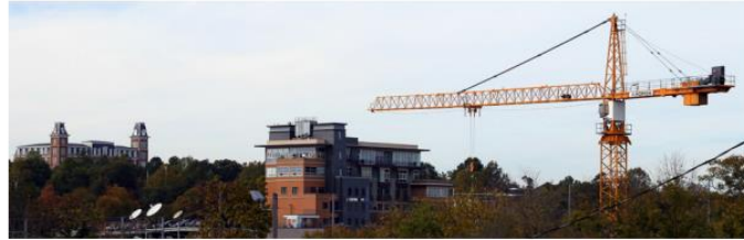
Photo 3.8 - Construction in Downtown Fayetteville
