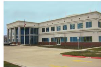
Photo 12.31 - Clean Technology Building
