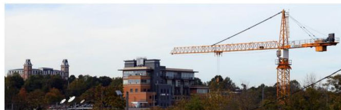
Photo 3.8 - Construction in Downtown Fayetteville
