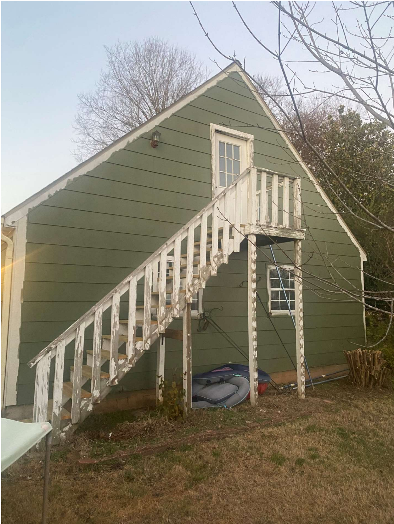
Elevation View of Exterior
