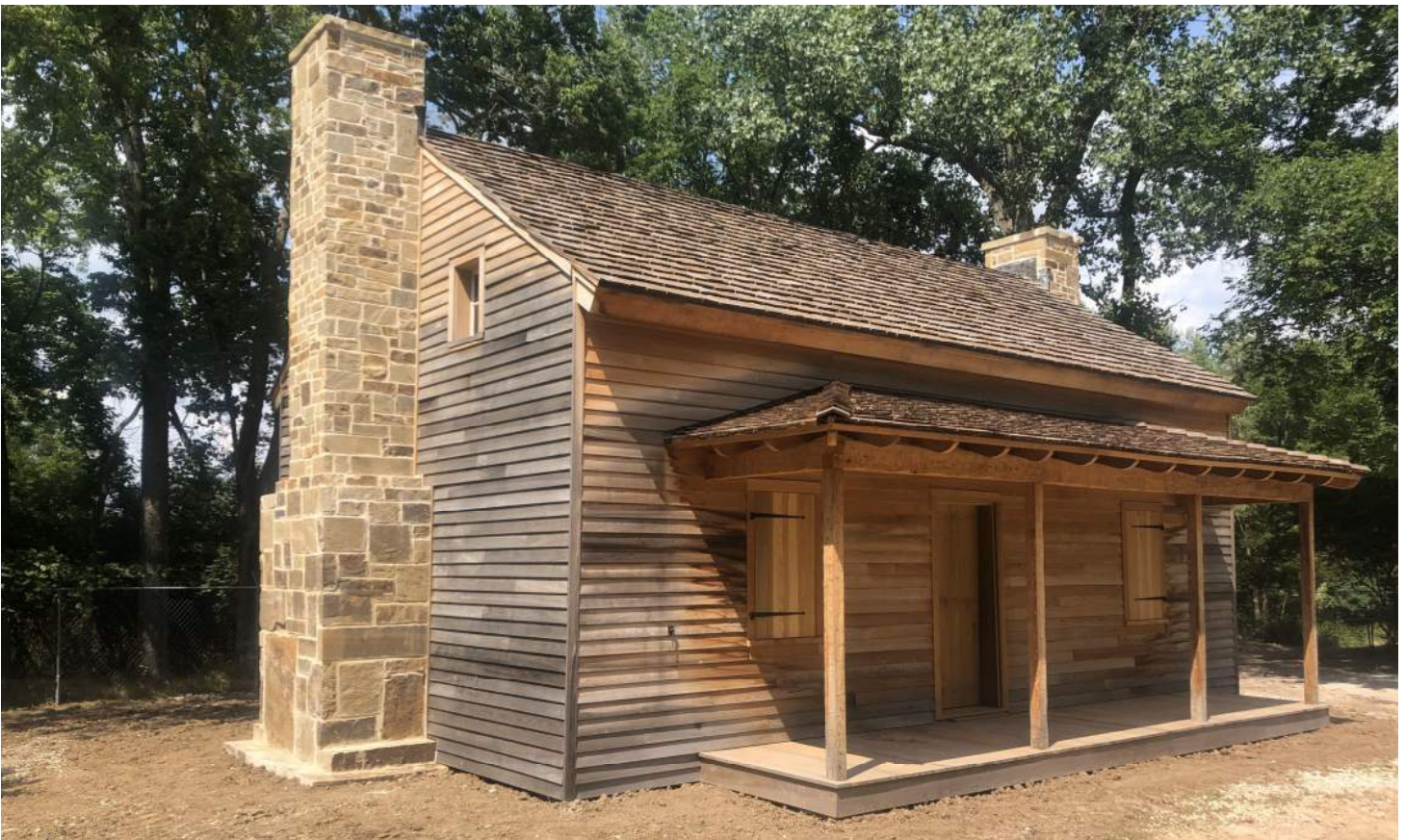
Woolsey Historic Homestead Renovation
