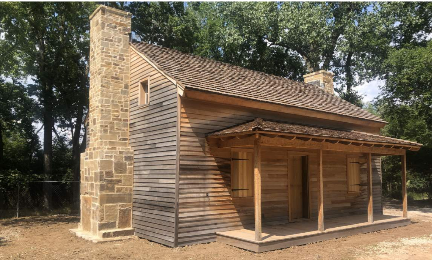
Woolsey Historic Homestead Renovation
