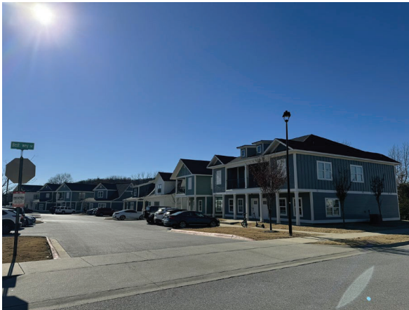
Primary improvements, looking south
