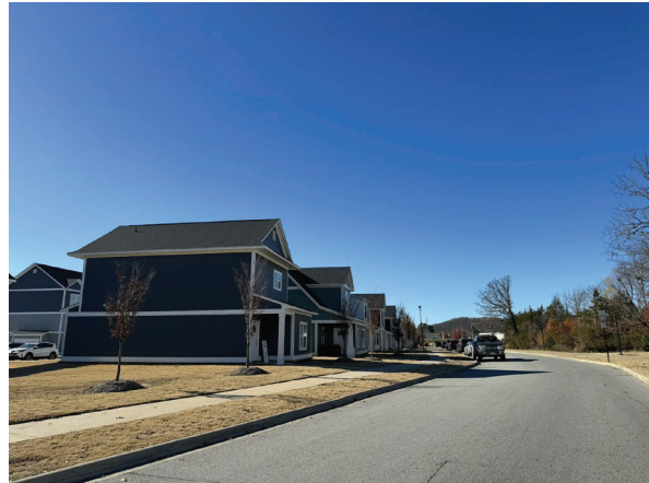
Subject frontage, looking west
