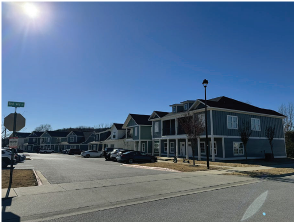
Primary improvements, looking south
