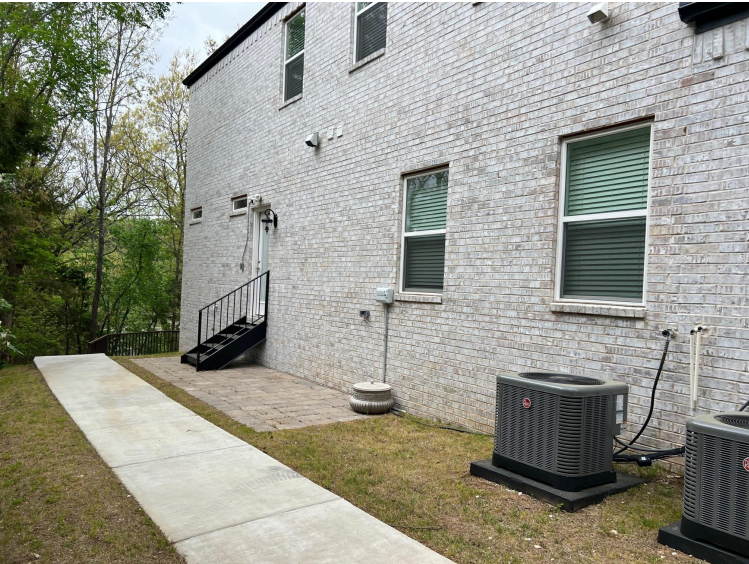
VIEW LOOKING PROJECT SITE
