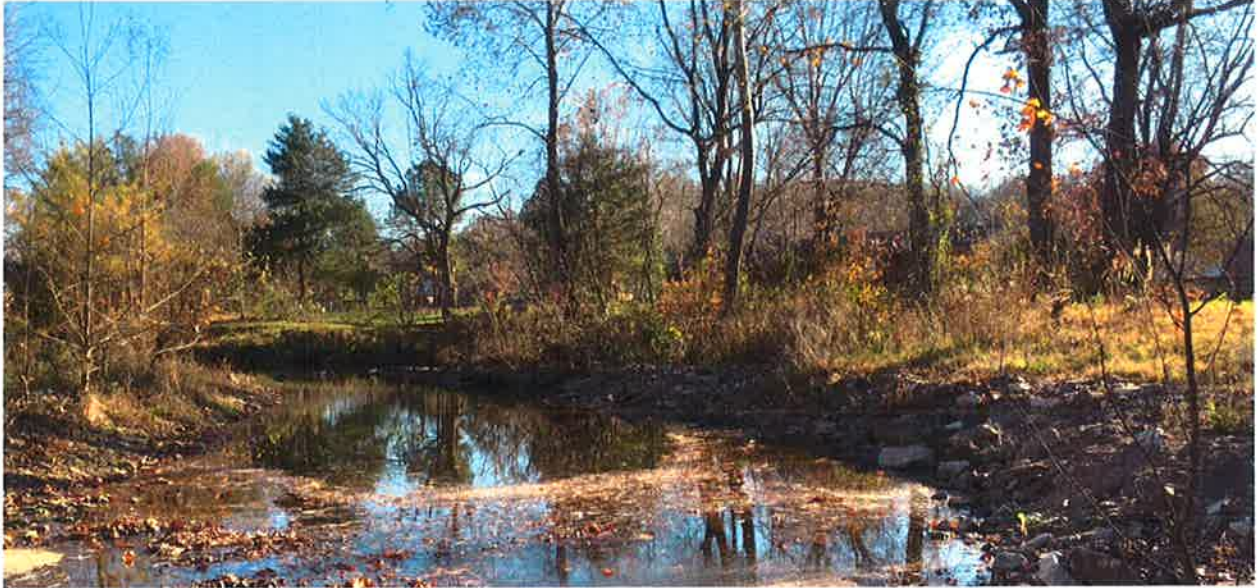
Figure 4 Temporary fill was placed along the scoured streambank of Niokaska Creek. The temporary fill will mobilize and be washed away from the scoured area that is protected by this short-term and temporary effort.
