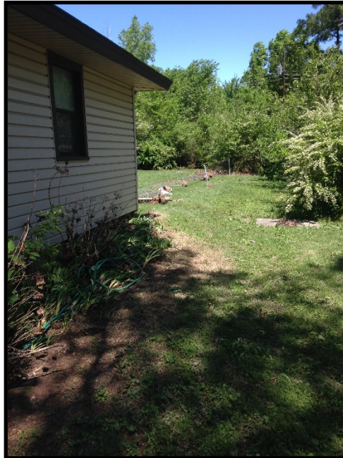
Fence Damage Valley Drive
