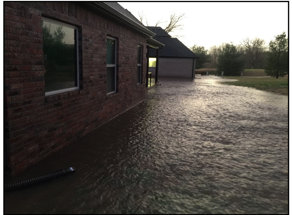
E Spyglass Hill Property Flooding
