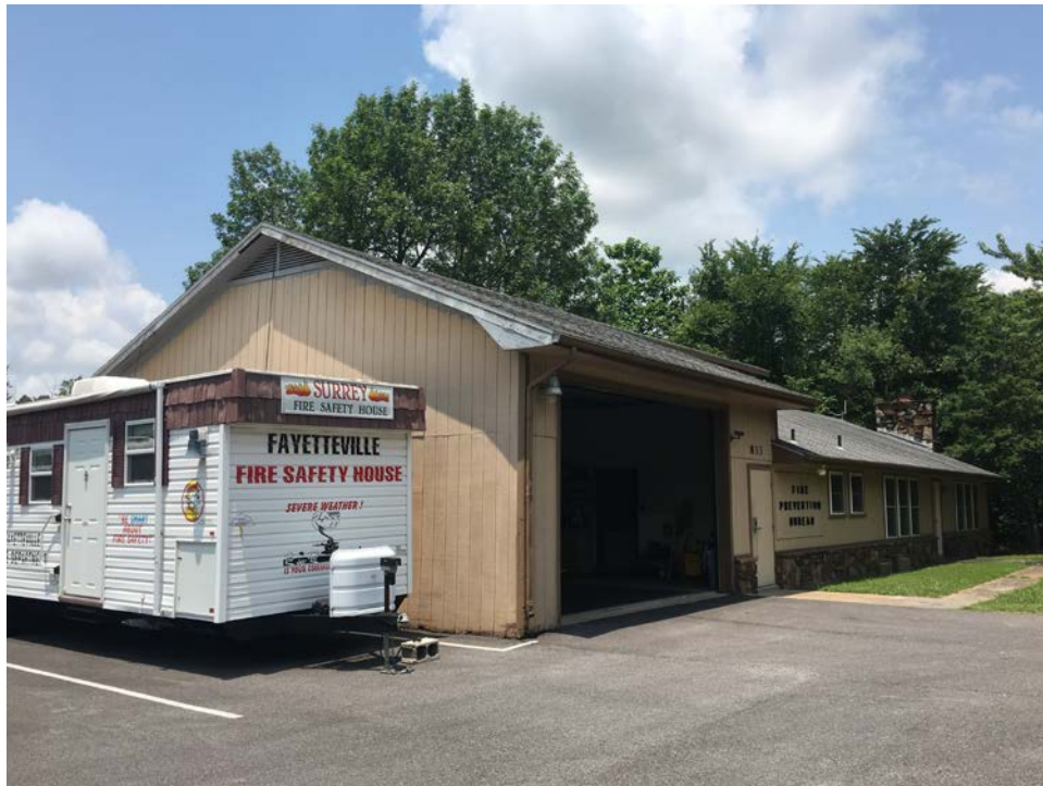
SOUTH AND EAST SIDES OF SUBJECT BUILDING – LOOKING NORTHWESTERLY
