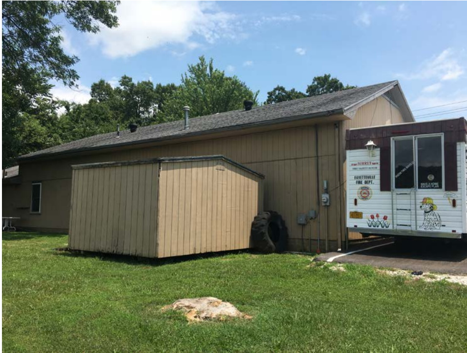
WEST SIDE OF SUBJECT BUILDING AND STORAGE SHED – LOOKING NORTHEASTERLY
