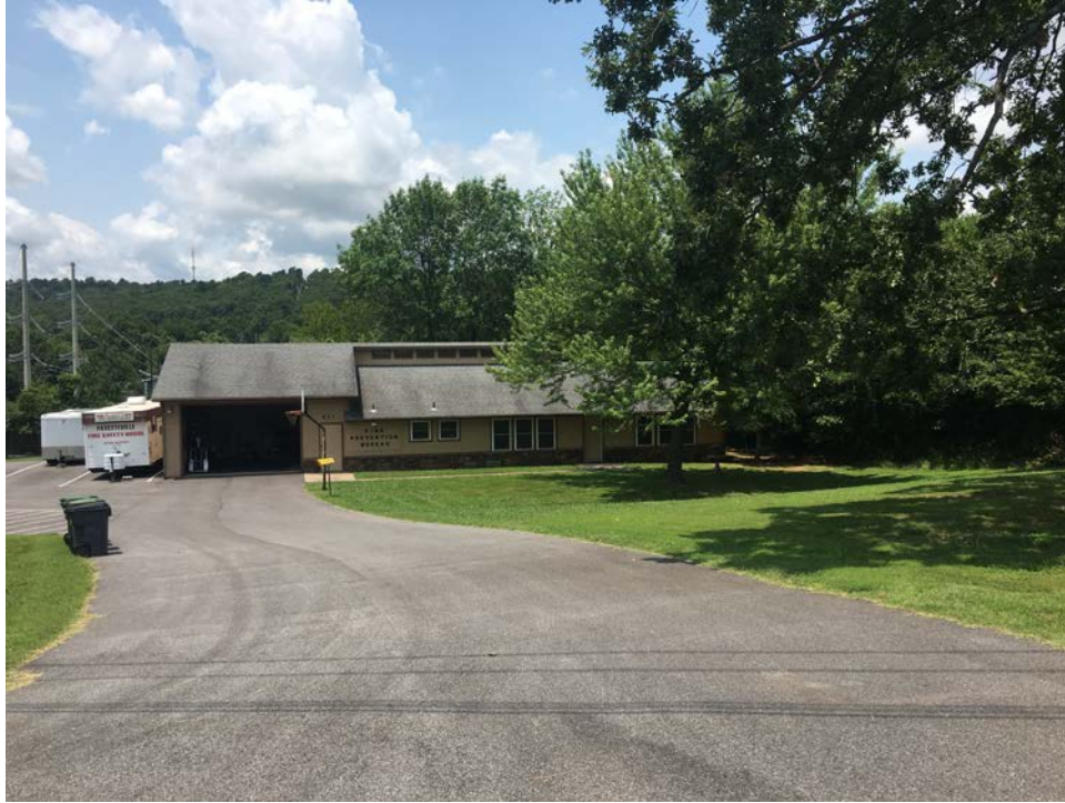
EAST SIDE SUBJECT BUILDING – LOOKING WESTERLY
