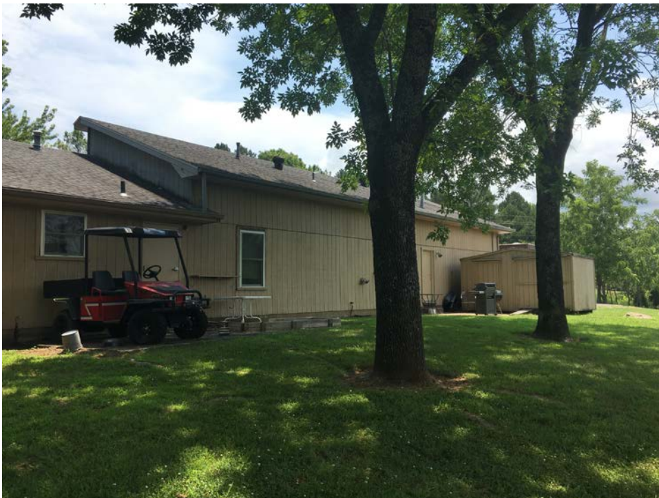
WEST SIDE OF SUBJECT BUILDING – LOOKING SOUTHEASTERLY
