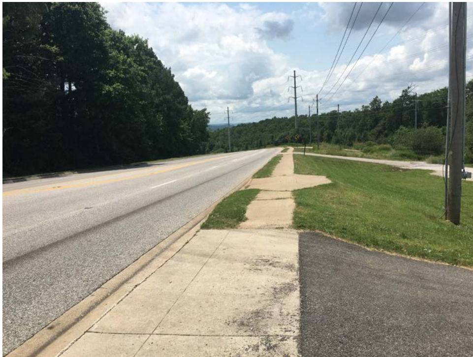
NORTH CROSSOVER ROAD – LOOKING SOUTHERLY
