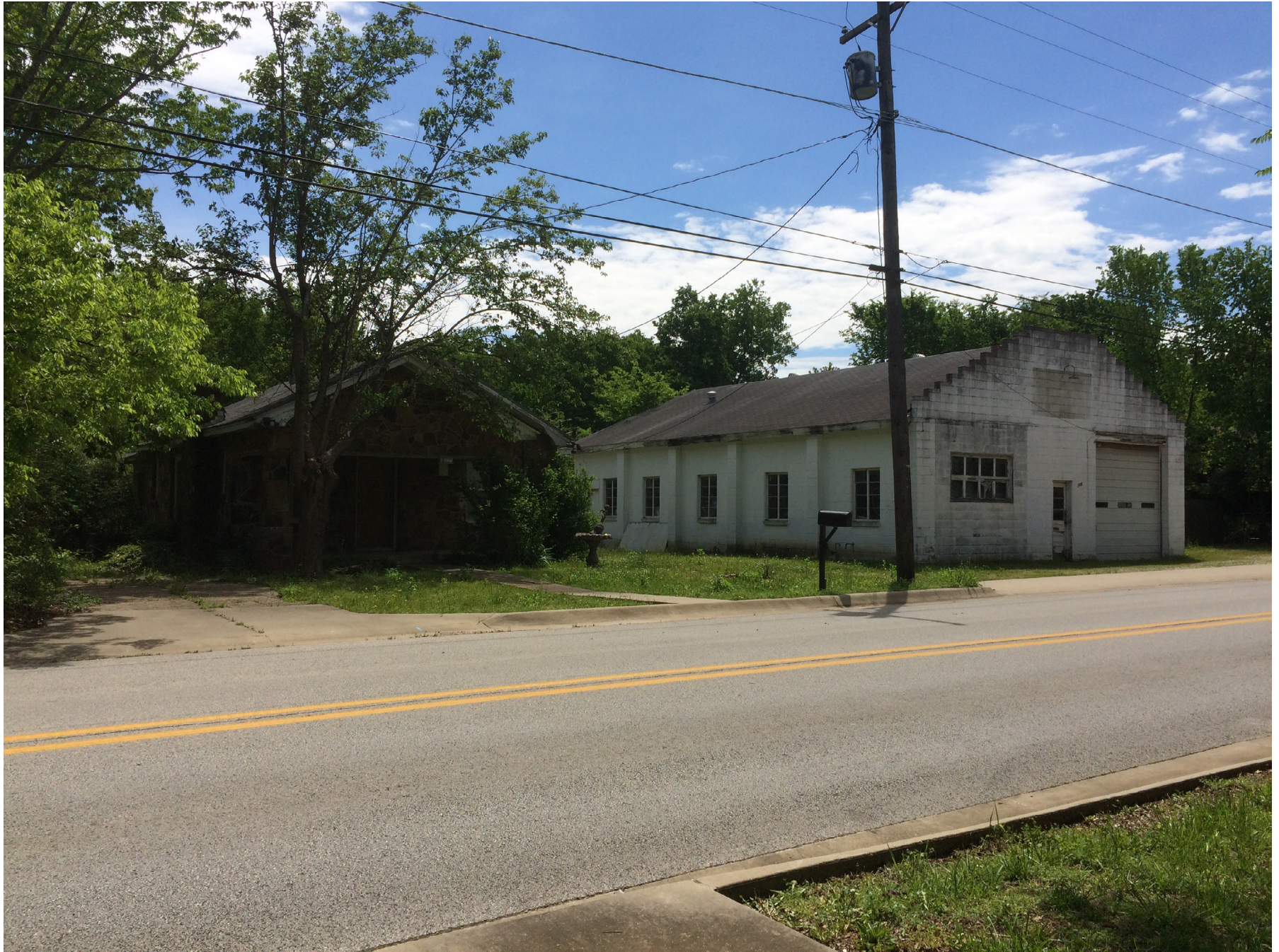
11. Staff Photo - 17-5770 RZN - Looking at 708 & 710 S College from Walker Park; Across alley ROW from rezone
