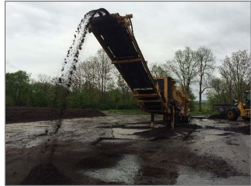
Picture 6-5: Screening Finished Compost
