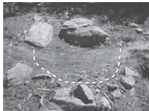
Knicks are constructed into existing trail tread in order to drain puddles from flat areas.
