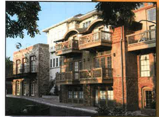
Three Sisters Building
