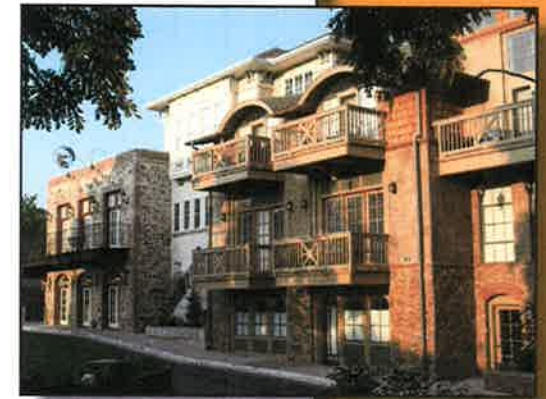
Three Sisters Building
