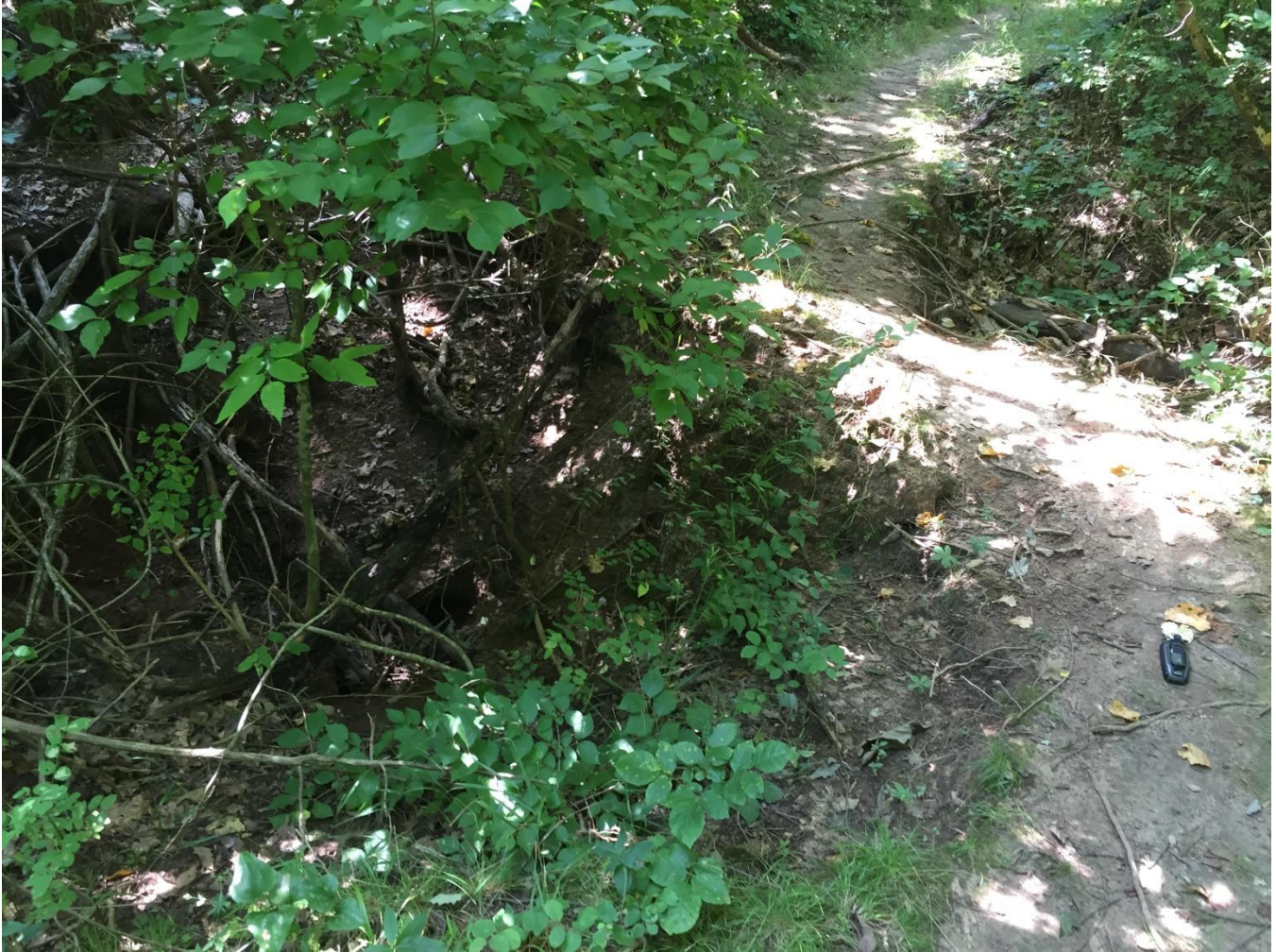
11. Heavy erosion/sinkhole on both sides of Crazy Mary Trail. Facing south 180°.
