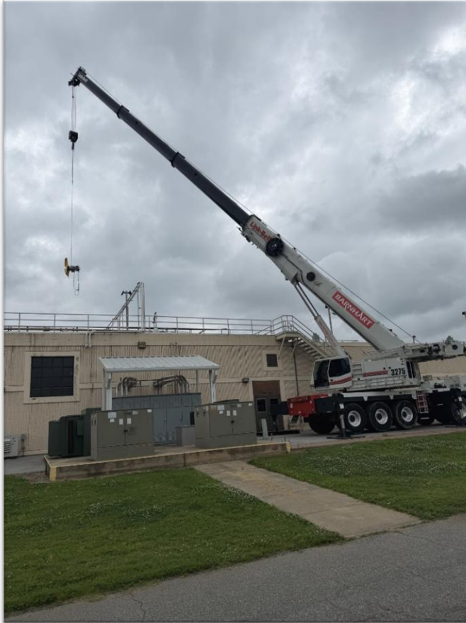
*Pictured above: mixer replacement
