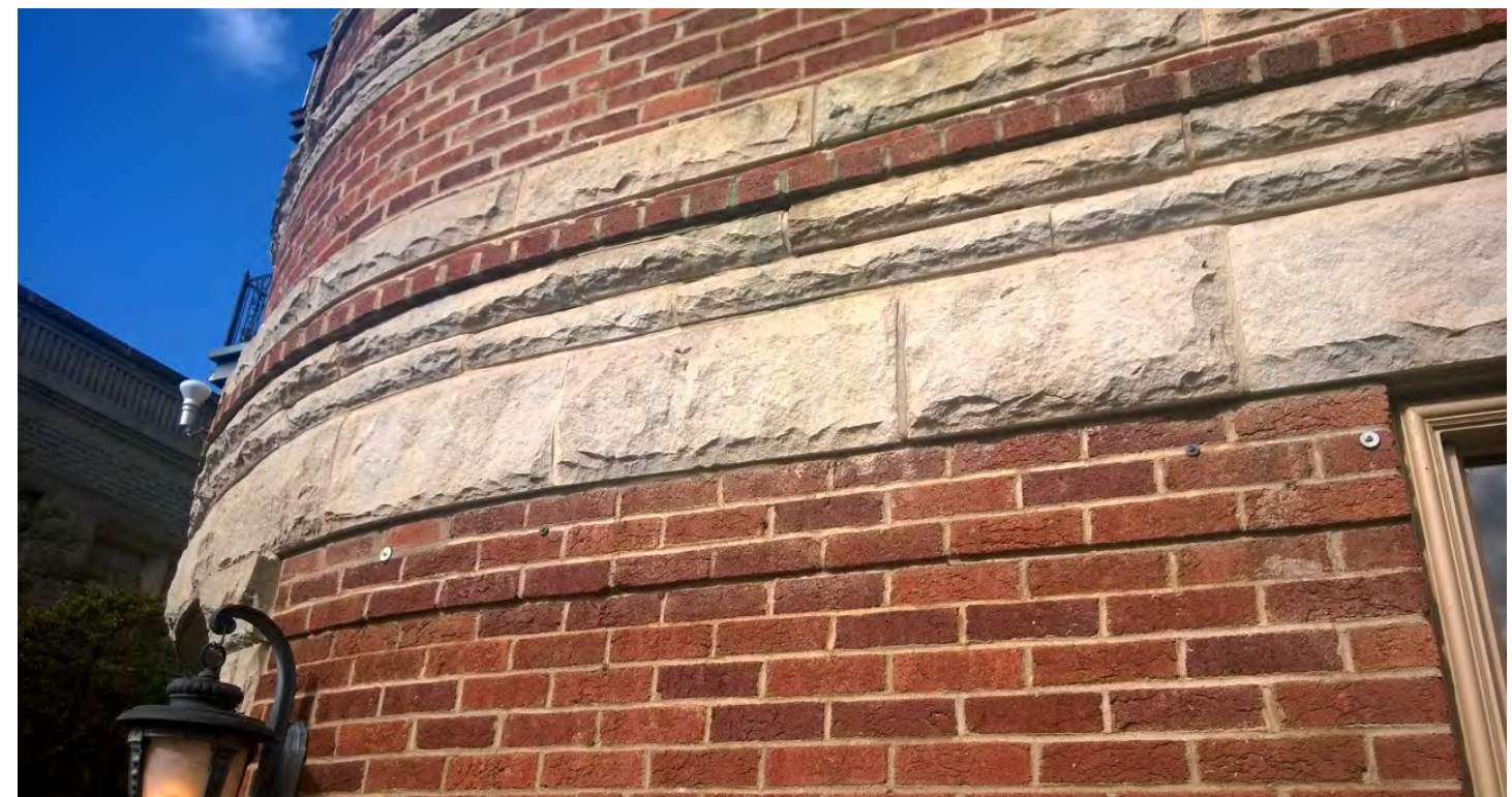
THREE SISTERS BUILDING
