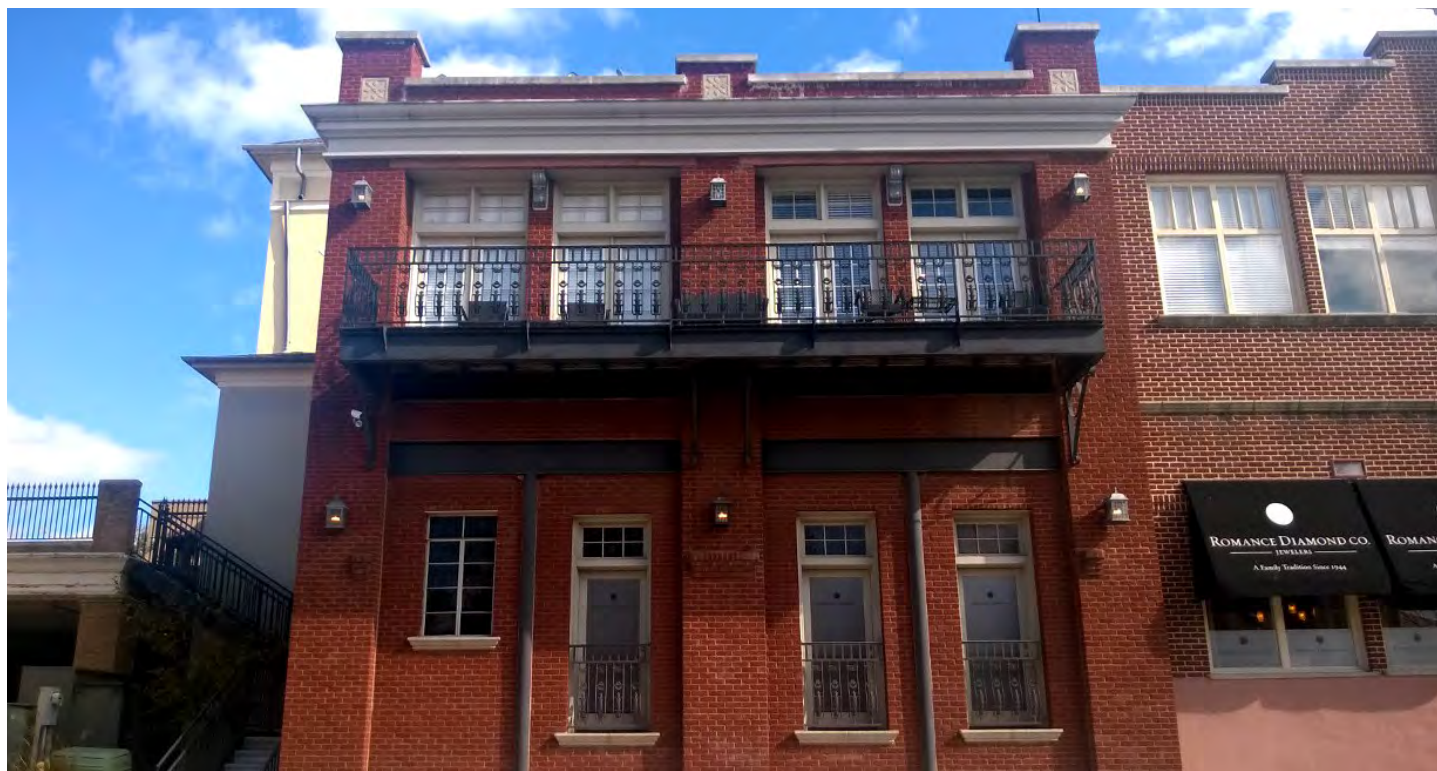
THREE SISTERS BUILDING
