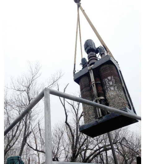
Crane removing Channel Monster for repair.
