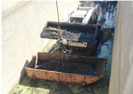
Cleaning grit out of the south contact basin.
