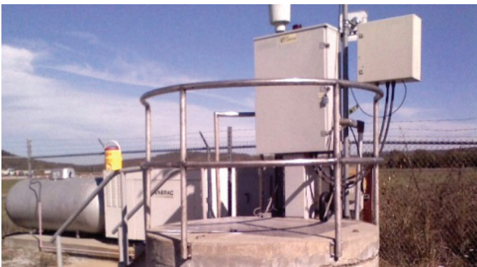
New safety rails at Airport East Lift Station (LS 24).
