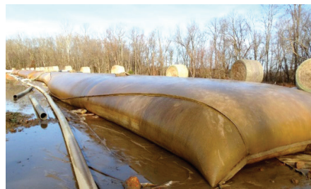
Geobag after being filled with sediment slurry allowing excess water to escape, a process called "dewatering".
