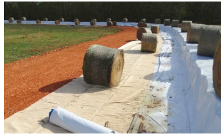
Geobags deployed with round bale containment berm.
