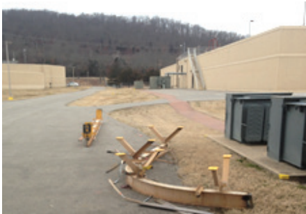
Old chlorine hoist and rails.
