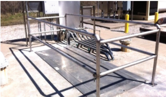
New safety rails at Mally Wagon Lift Station (LS 19).
