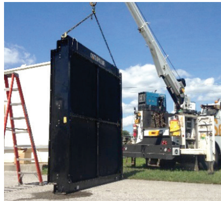
Crane removing radiator for repair.
