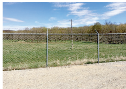
View looking south from Noland after flooding.
