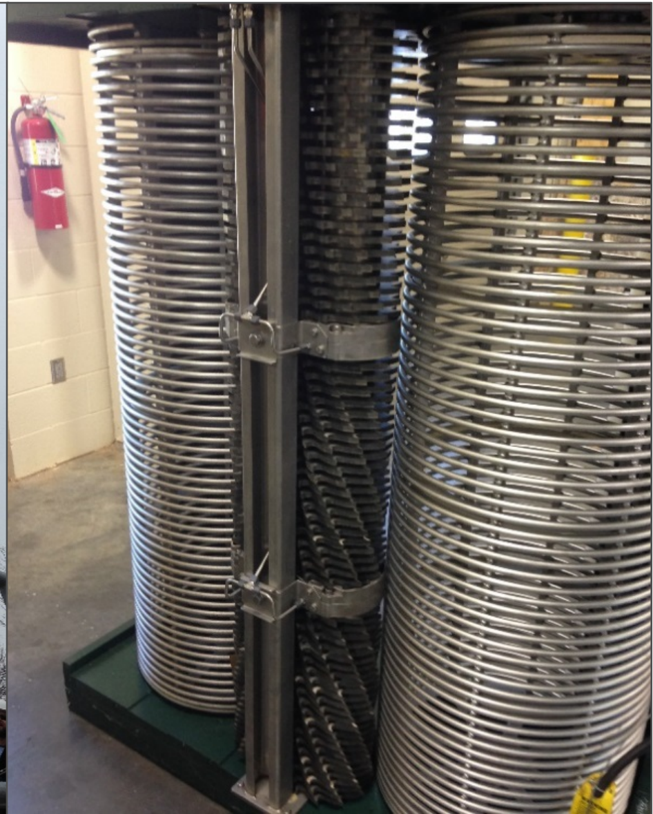
After Clean Up
