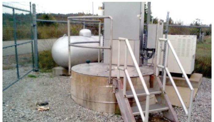
New safety rails at Airport South Lift Station (LS 34).
