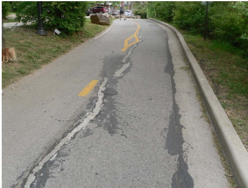
Existing Trail Condition – looking south toward Maple Street
