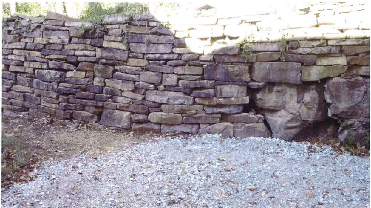
Representative Wall Section with Dry Stacked Rocks and Existing Rock Embankment
