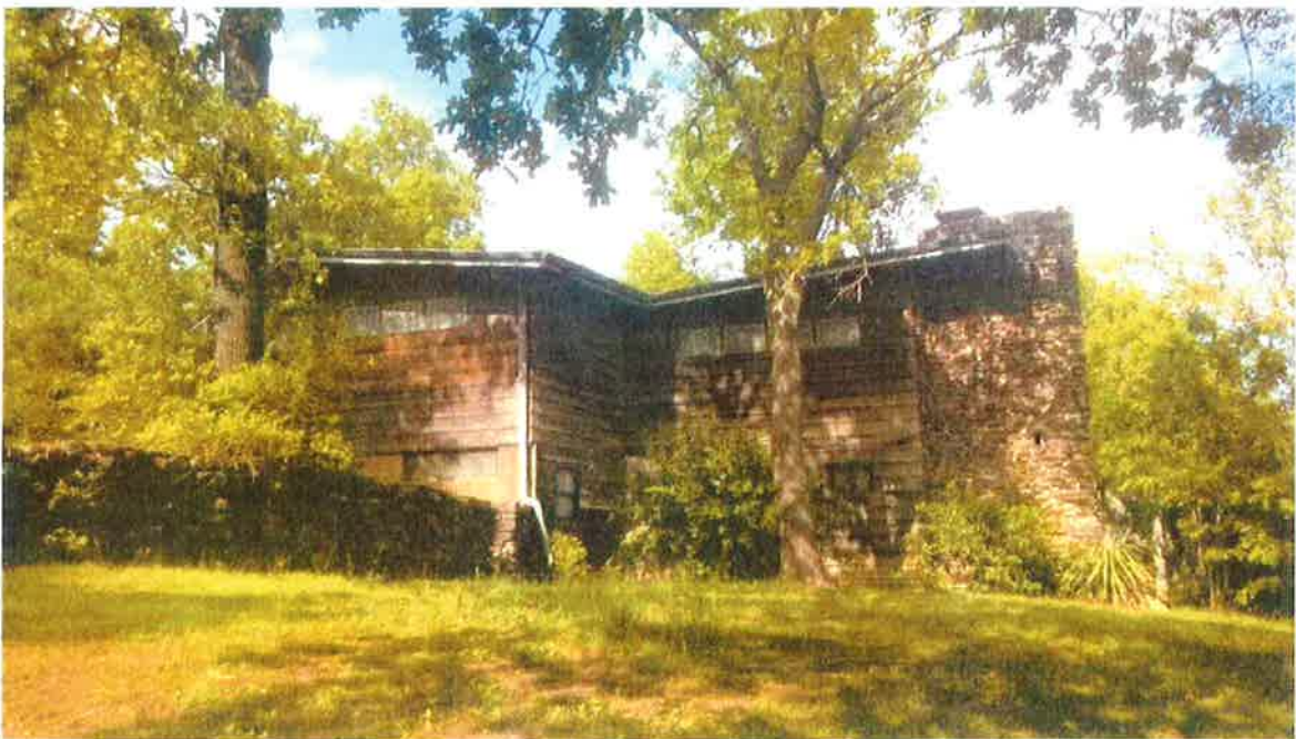
HORNSBY EXISTING HOUSES
