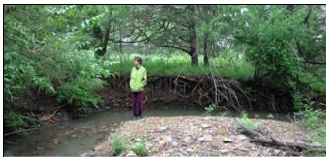
Figure 3 Erosion on Unnamed Tributary to Cato Springs
