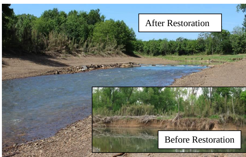
Figure 2 WFWR restoration at Fayetteville Municipal Airport
