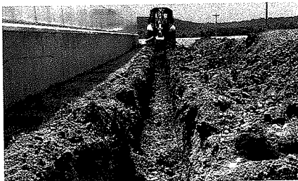
Trench for vapor phase piping
