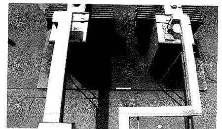
Recently installed protective covers
