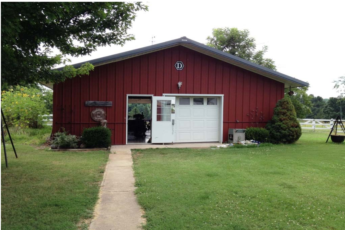
NORTHWESTERN ELEVATION OF SHOP BUILDING LOOKING SOUTHEASTERLY
