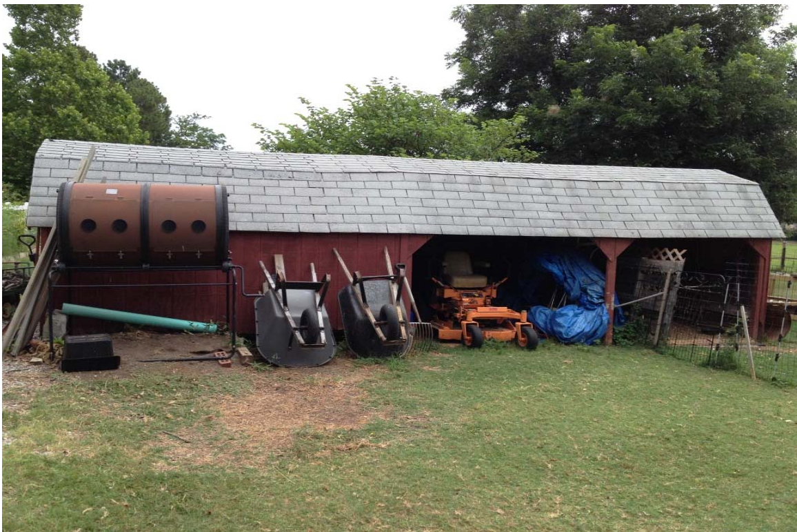
VIEW OF SHED AT 2648 OLD WIRE ROAD
