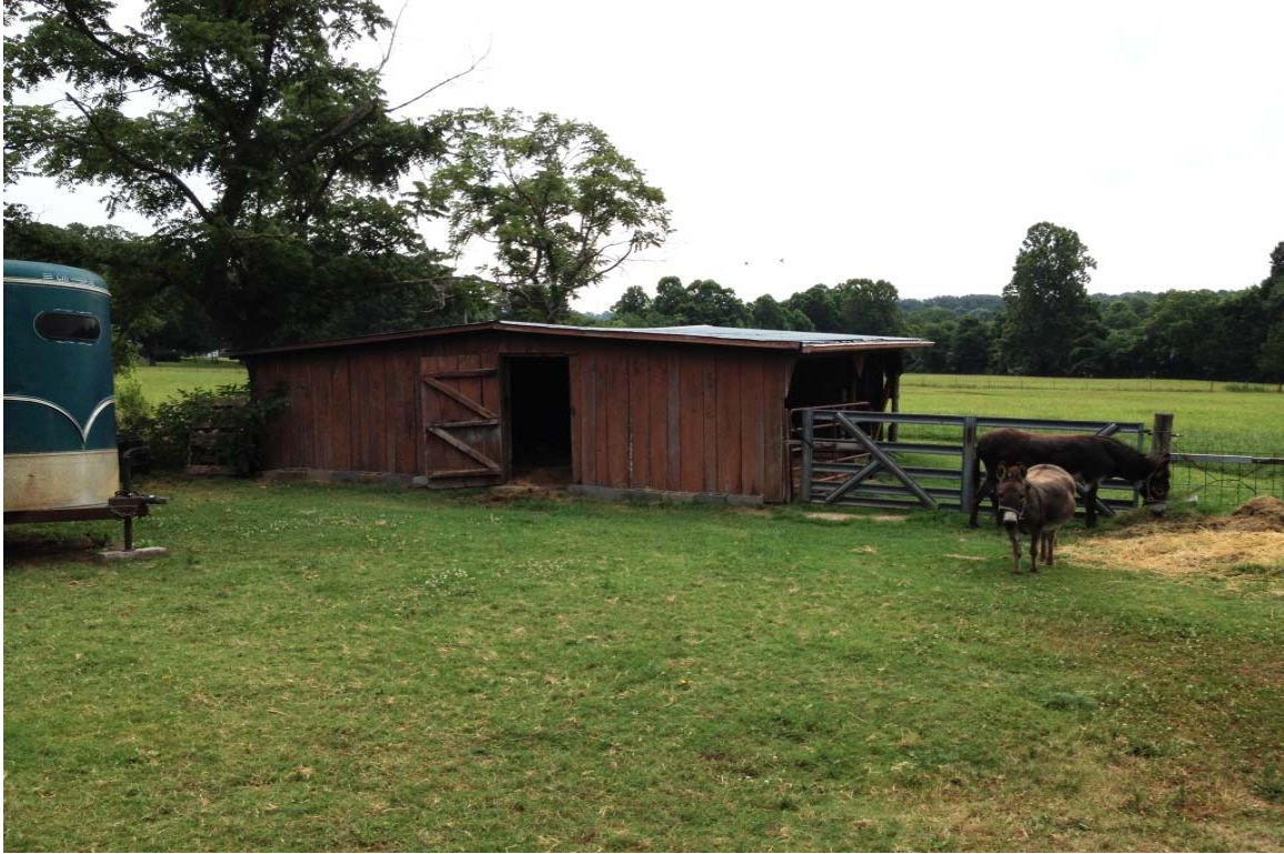
VIEW OF SHED AT 2648 OLD WIRE ROAD
