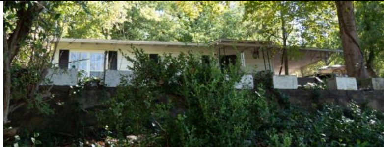
Photo by Post Oak Preservation Solutions
