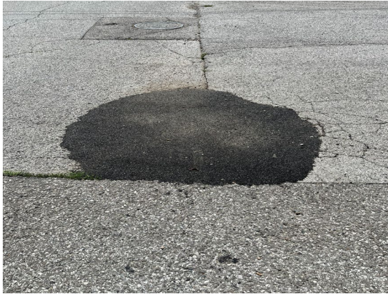
Picture 3: Typical Pothole Repair
