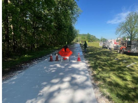
Picture 8: Hamstring Trail Asphalt Replacement
