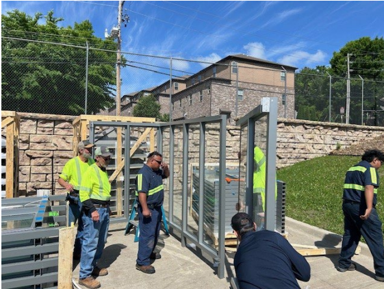
Picture 23: Bus Shelter Assembly (1)
