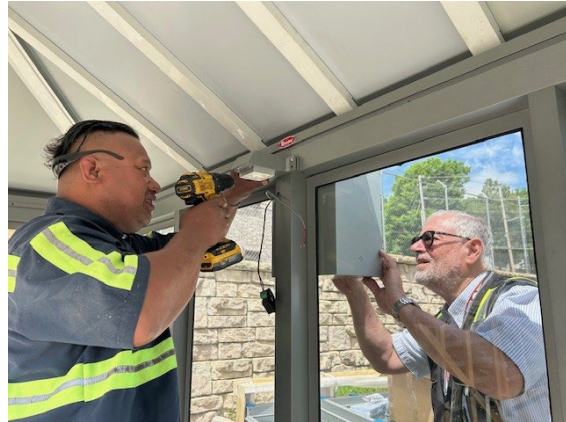
Picture 24: Bus Shelter Assembly (2)
