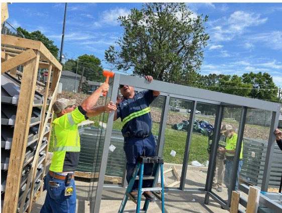
Picture 25: Bus Shelter Assembly (3)
