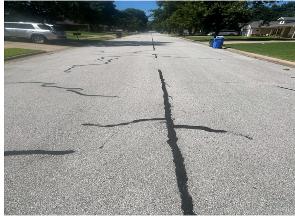
Picture 4: Crack Sealing
