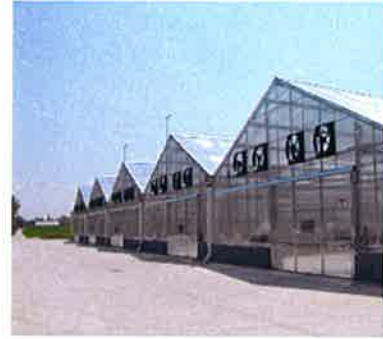
The new biosolids solar dryers
