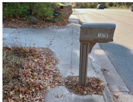
Multiple mailboxes obstructing sidewalk
