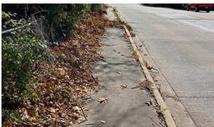
Debris & vegetation obstructing sidewalk
