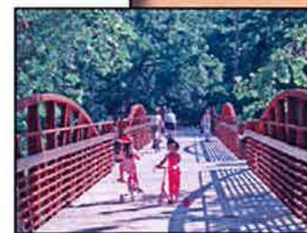
Lake Fayetteville Spillway Bridge
