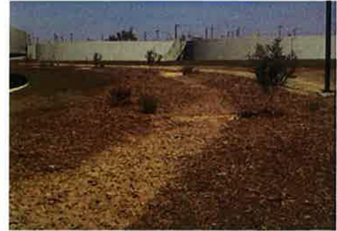
Erosion Control at West Side WWTP
