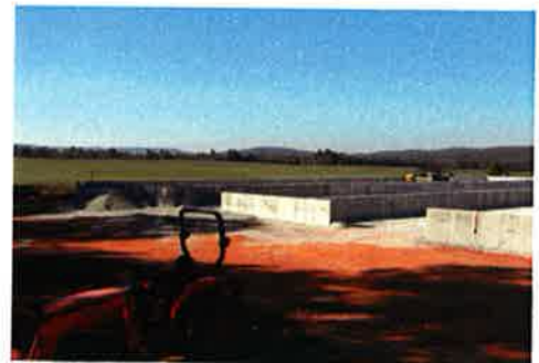
The new biosolids solar dryers' construction site
