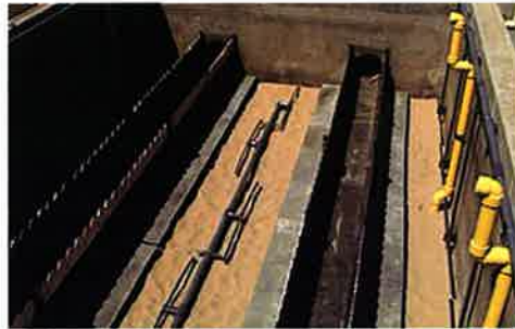
Filter cell rehab with new piping, baffle, and sand.
