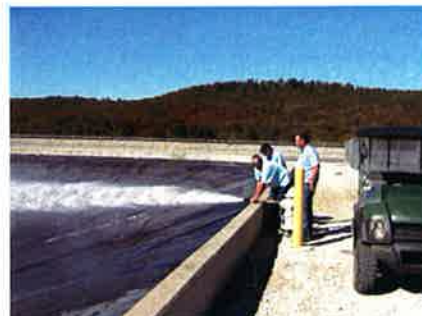
Installation of the new water canon at the influent storage pond
