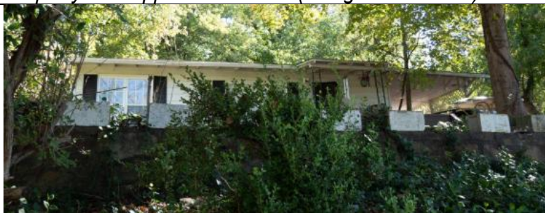
Photo by Post Oak Preservation Solutions
