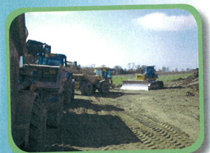
soil compaction during construction
