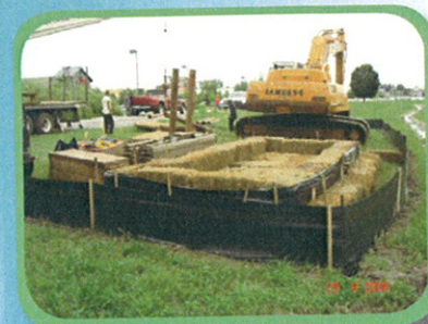
sediment filter used during construction
