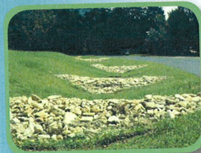
check dams slow water flow in swale
