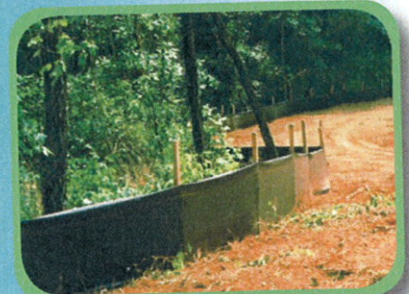
silt fence along construction zone
