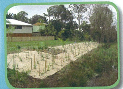
streambank restoration using landscape fabric
