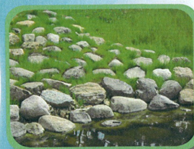
drainage riprap along streamside
