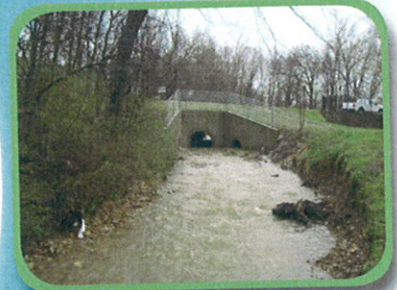
flood waters and streambank erosion
