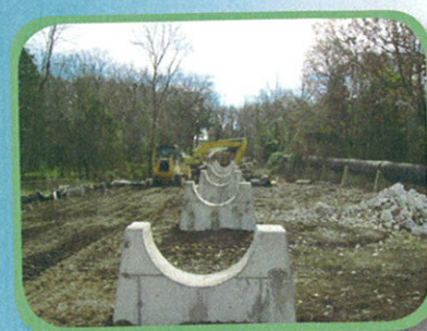
above grade piers outside of stream
