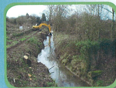
dredging of stream channel
