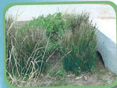
stormwater diffusion with plant materials
