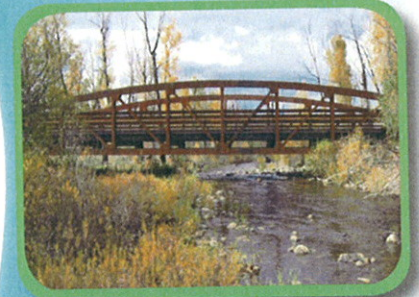
streamside low impact bridge
