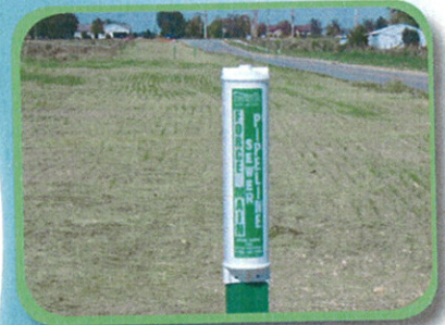
clearly labeled utility
