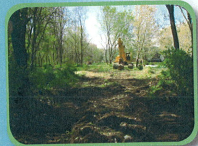
minimized utility easement work width
