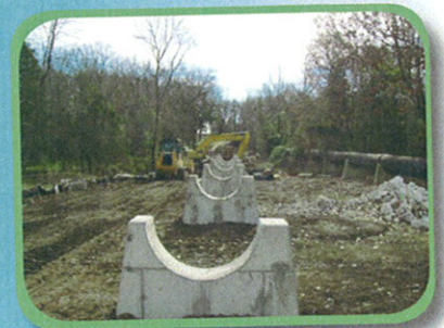
above grade piers outside of stream
