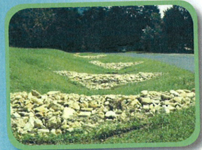
check dams slow water flow in swale
