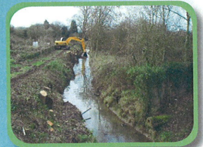
dredging of stream channel
