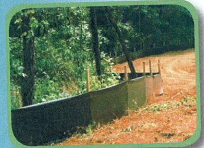
silt fence along construction zone
