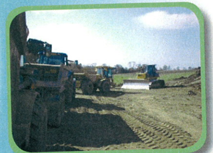
soil compaction during construction
