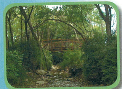
clear span trail bridge
