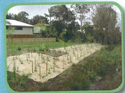
streambank restoration using landscape fabric
