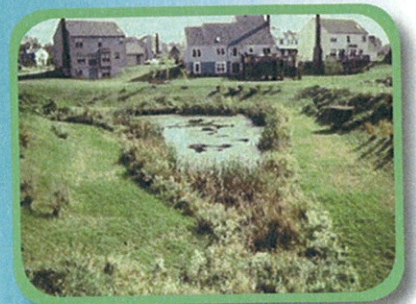
enhanced dry detention in residential neighborhood
