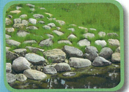
drainage riprap along streamside
