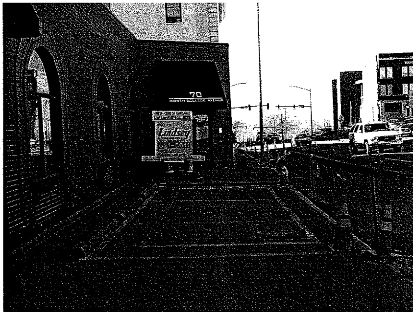
Concrete has been removed along the existing right-of-way.
