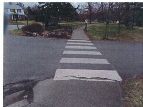
Existing entry on north side of Wilson Park on Prospect Street facing east
