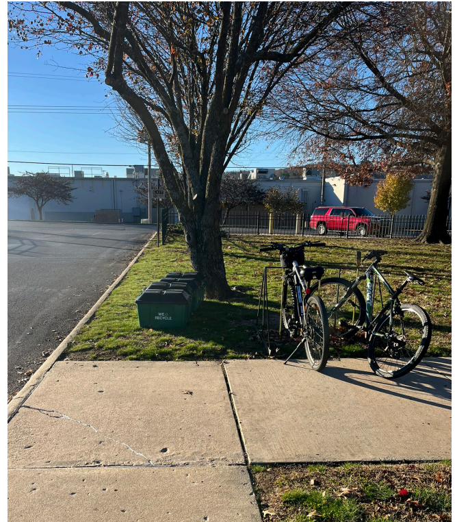
IMAGE 7.9 This bike rack style does not support bicycles properly. Replacement is recommended.
