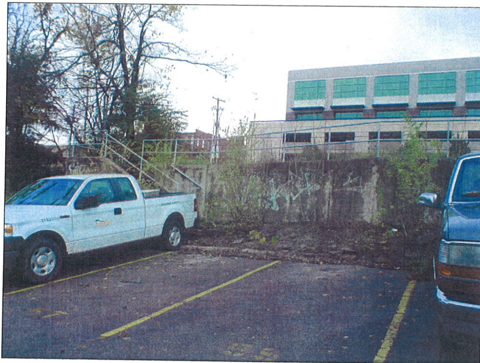
Railing and Stairs of Subject Looking North
