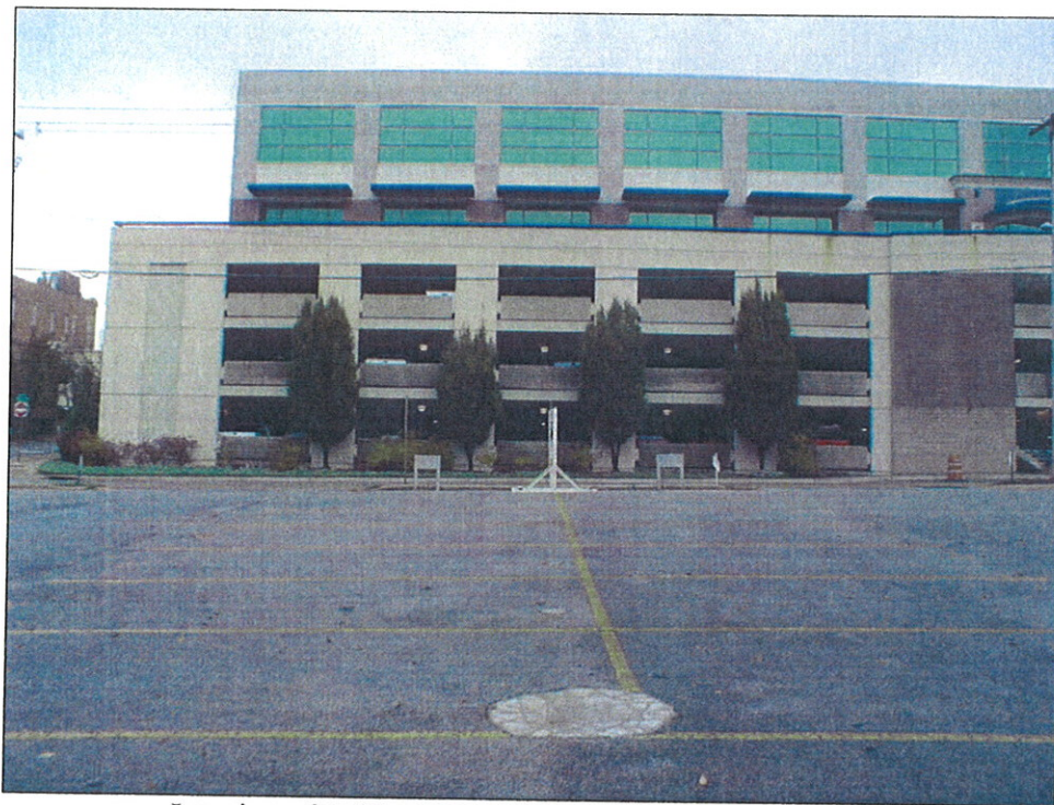
Interior of Subject Site Upper Level Looking North
