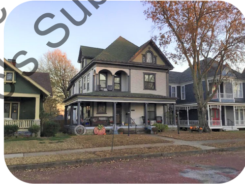
Historic Resources Survey Update of the Belle Grove NRHP District Fort Smith
