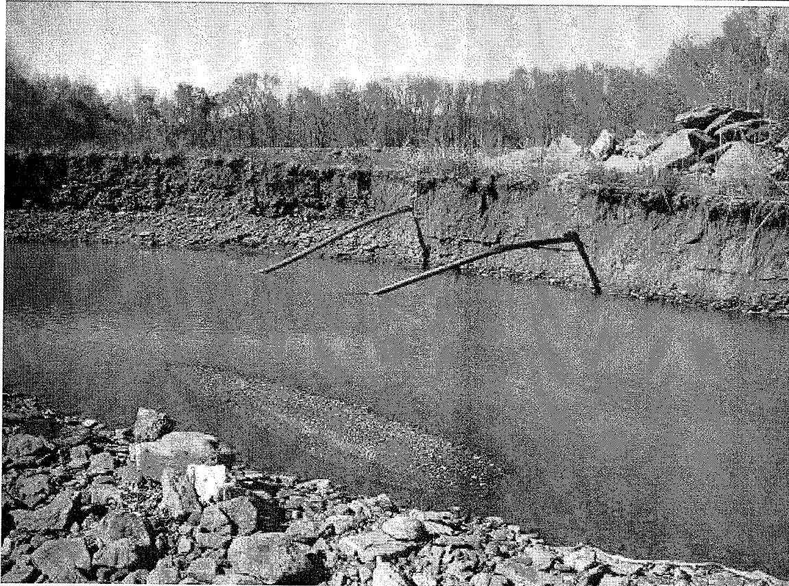
Figure A4-01 Typical site conditions of the WFWR at Brentwood prior to restoration. Photo on the bottom shows a streambank that was eroding an average of 13 ft/yr for typical flow years.
