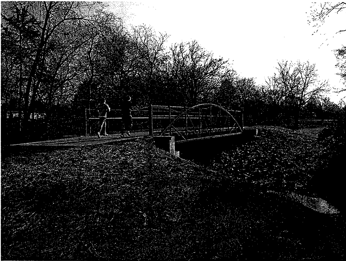
50' long Town Branch Creek Bridge near the intersection of Razorback and 15 th .
