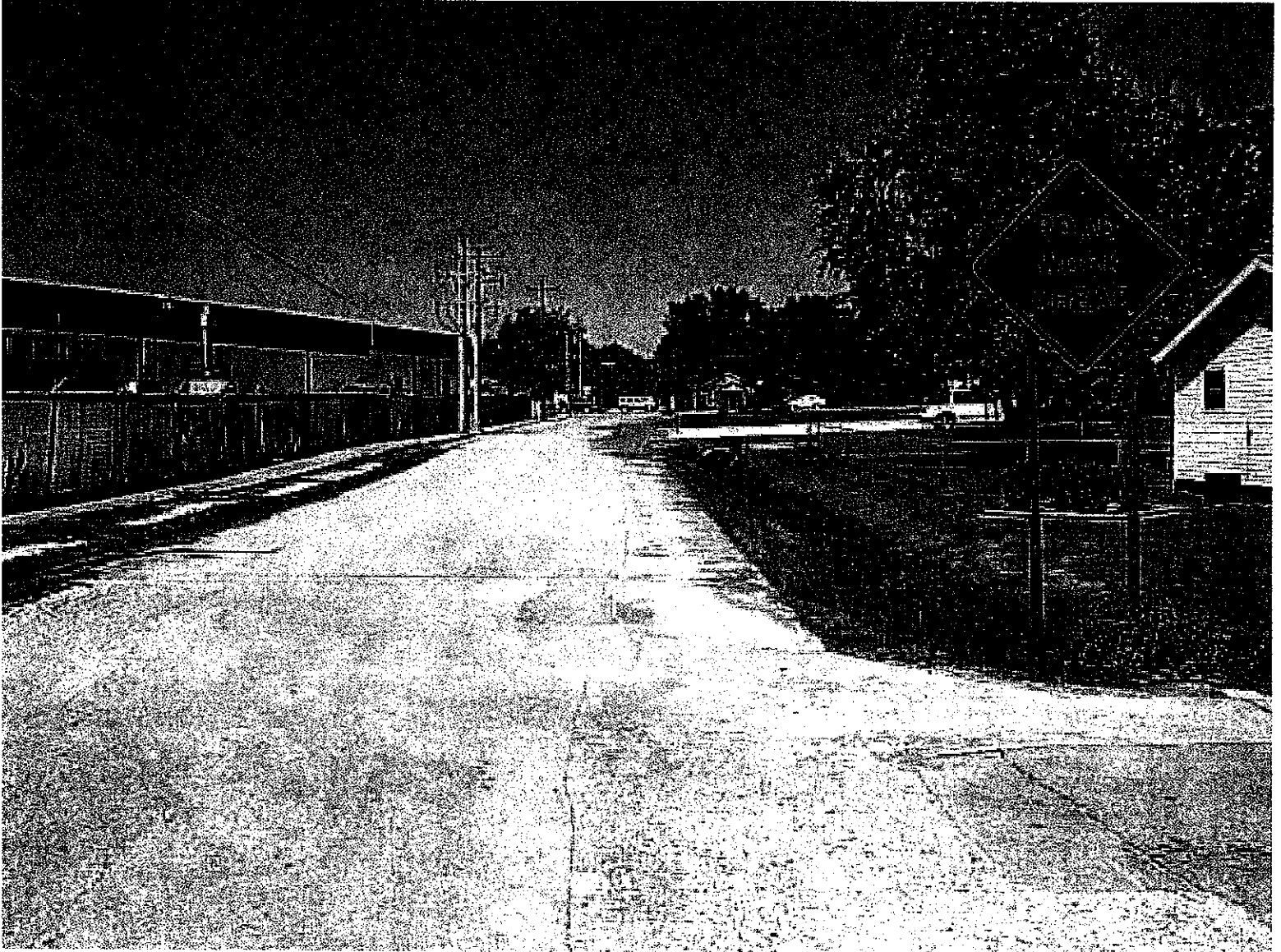
LEE/RAY - LOOKING NORTH (EAST SIDE)
