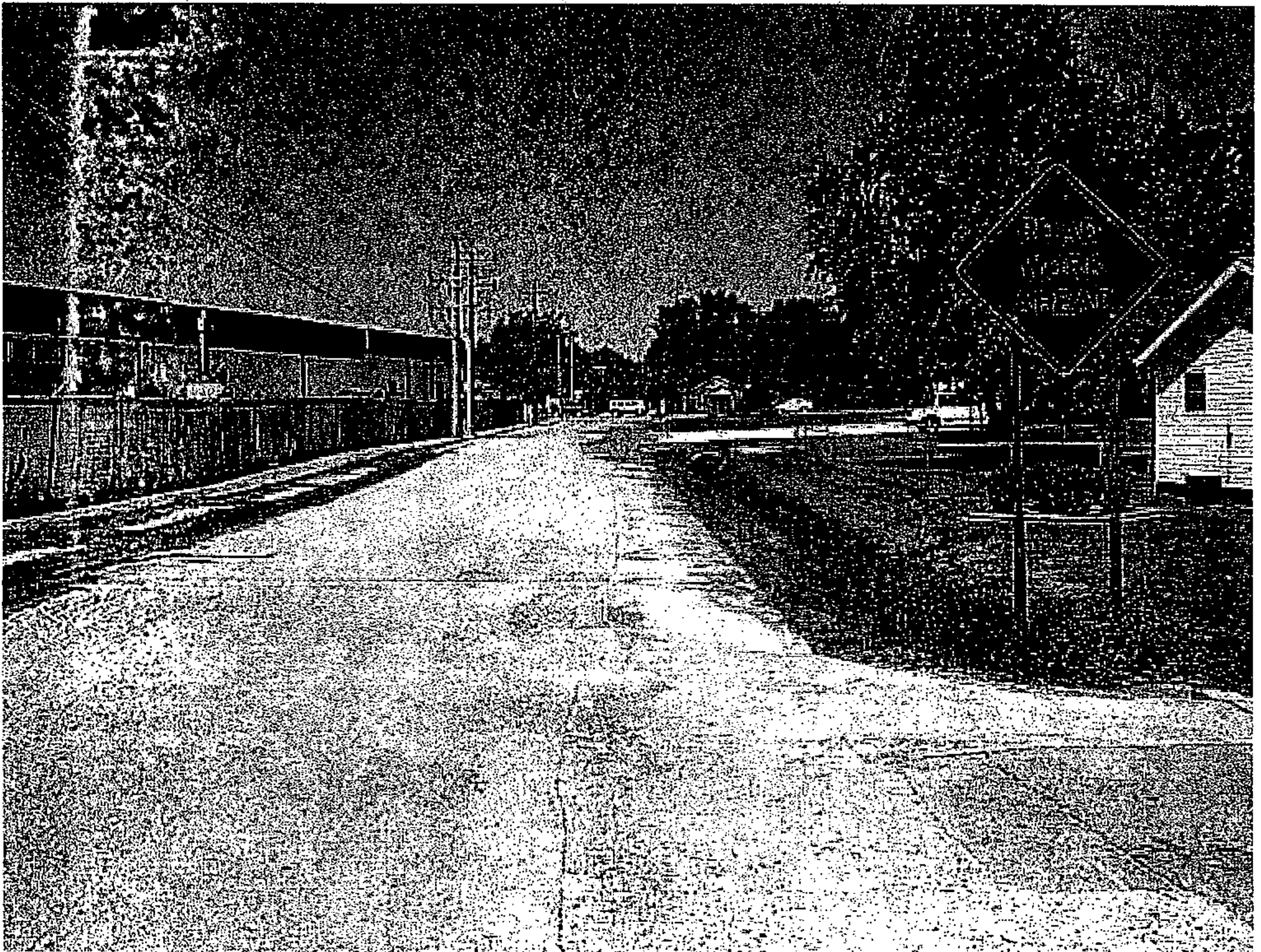
LEE/RAY - LOOKING NORTH (EAST SIDE)
