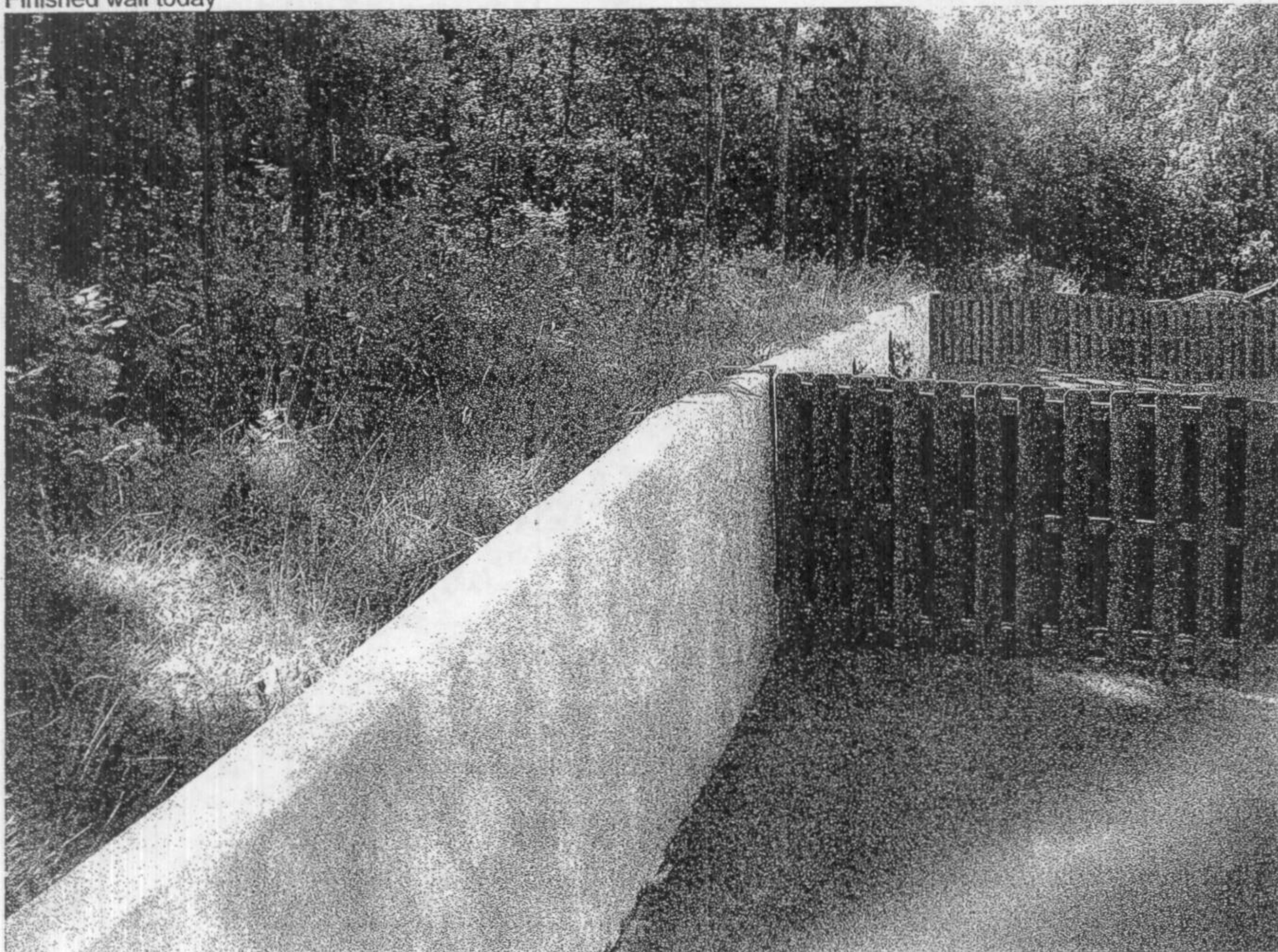
Finished wall today
